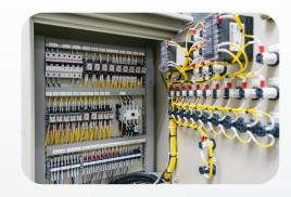
In a new installation, one twisted pair cable can replace all yellow control cables required prior to 10BASE-T1S
